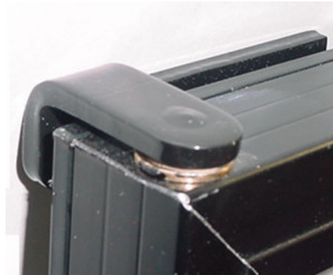
New hinge installed
